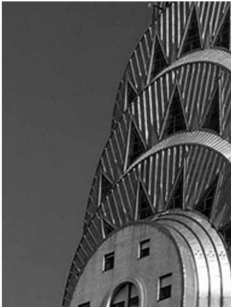
The pinnacle of New York's Chrysler Building is clad with type 302 stainless steel
