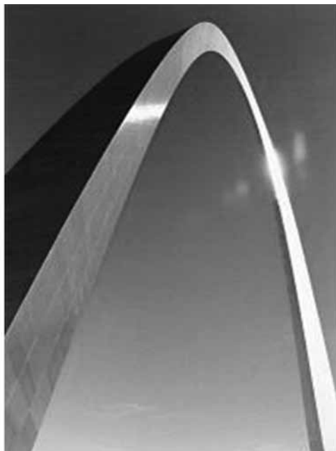
The 630-foot (192 m) high, stainless-clad (type 304) Gateway Arch defines St. Louis's skyline
